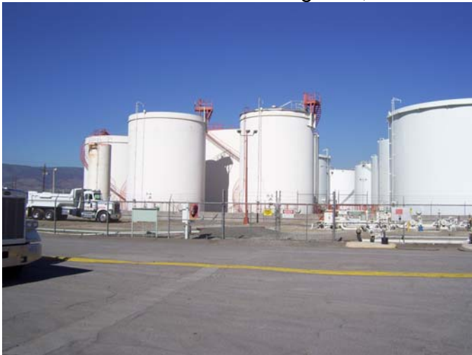
Sparks, Nevada Terminal
