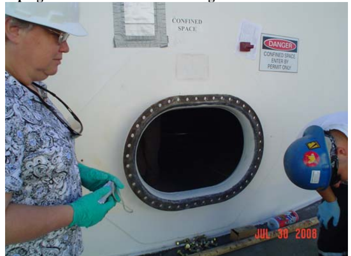
The entry to the inside of the tank
